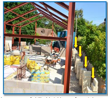
The stalwart gang of skilled bricklayers from John Loving's in Dorchester continue to work at a rapid pace and the walls are springing up to the first six-foot level all around the site. In our picture left we see the finishing touches applied to the outer wall of the block and beam floor under the chair store and office. The insulation panels are in place and pinned to the inner breezeblock wall. Then there is an air gap, to prevent damp transmission to the outer wall architectural blocks.
